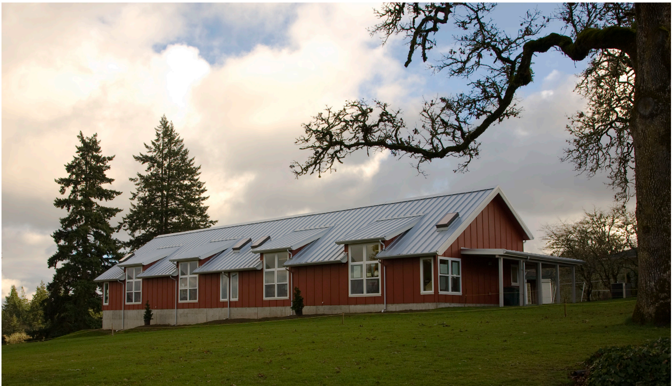
Oak Hill School's north-facing facade.
